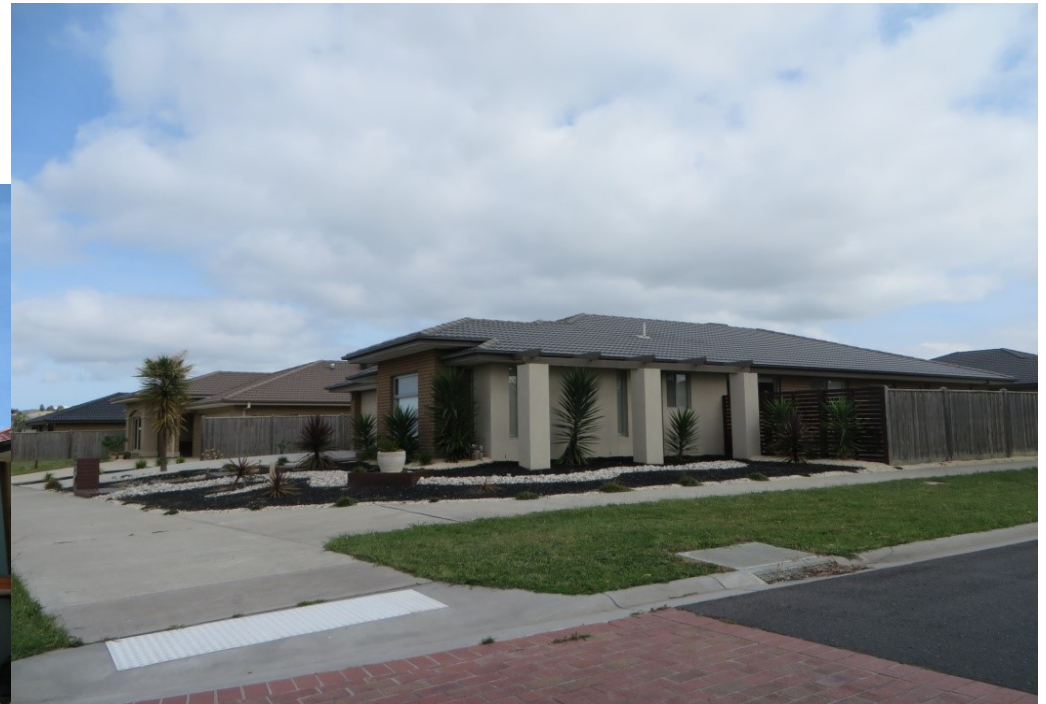
Vertical style windows matching the façade with feature piers
