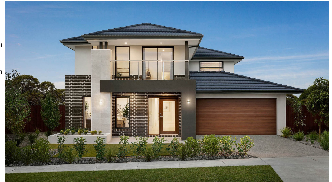
Contemporary Style Double Storey—Carlisle Homes— Bentley Facade
